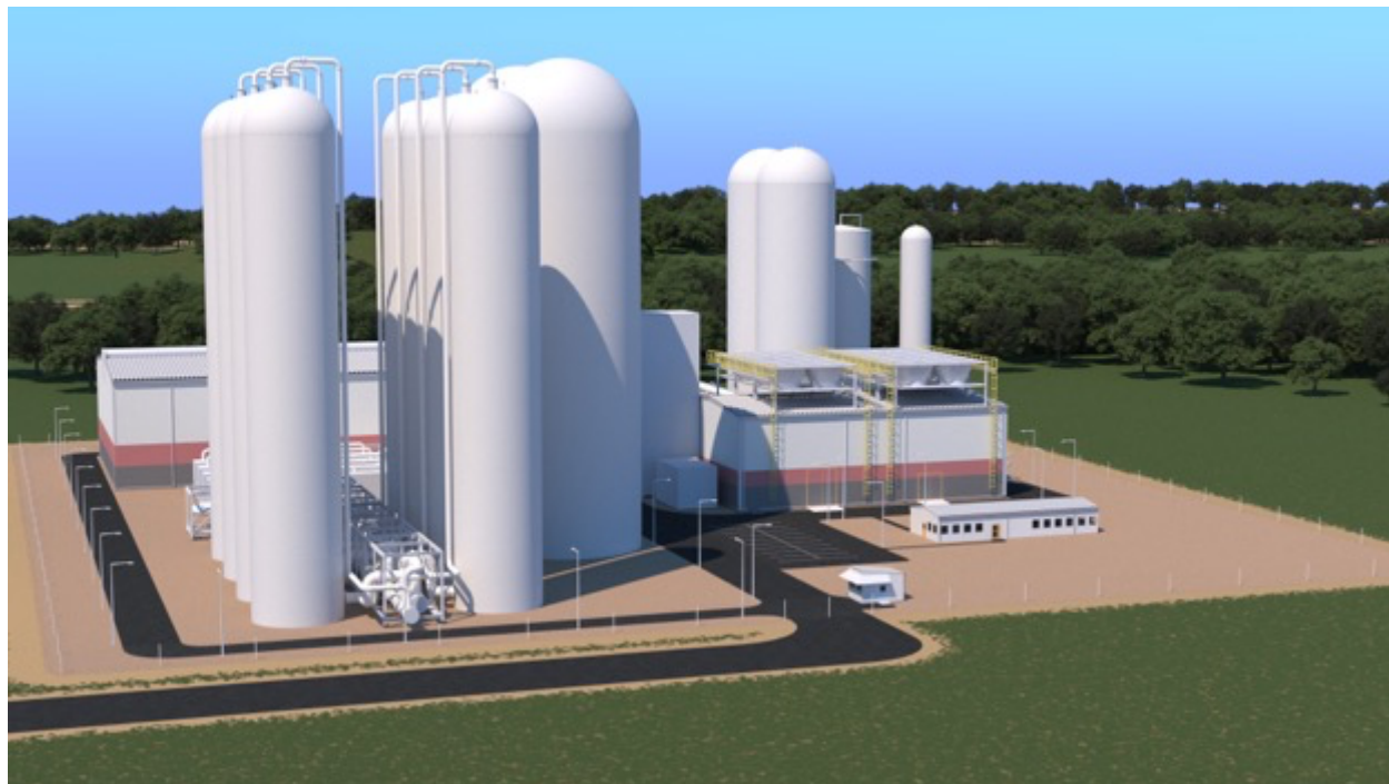
Fig. 2. 8 Liquid air storage as envisioned by Highview Power
